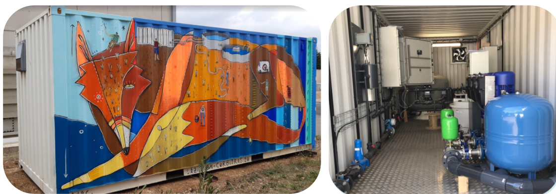
Figure 2 Pictures of a standard containerized 50 \text{m}^3/\text{h} REUSEbox.
