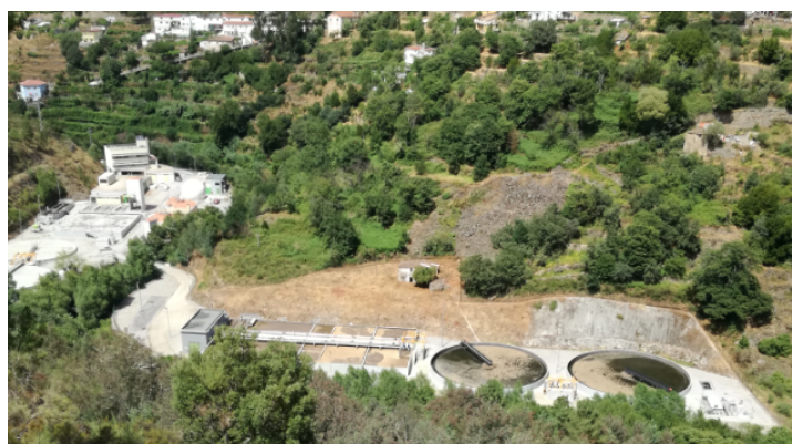
Figure 1 Aerial view of the entire extension of the Vila Real WWTP
