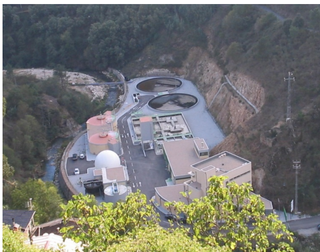
Figure 2 Second view of the part of the Vila Real WWTP
